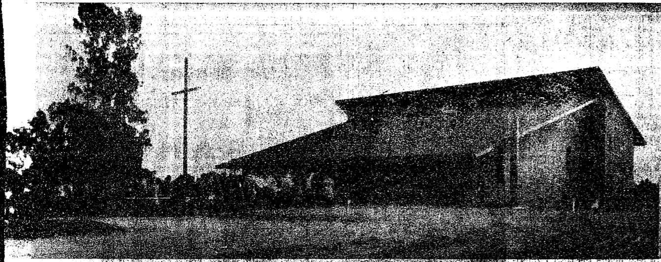
FAITH EVANGELICAL LUTHERAN CHURCH dedicated their new church Sunday, Sept. 24. Built at an actual cost of $175,000, much other work was donated by the congregation. A
